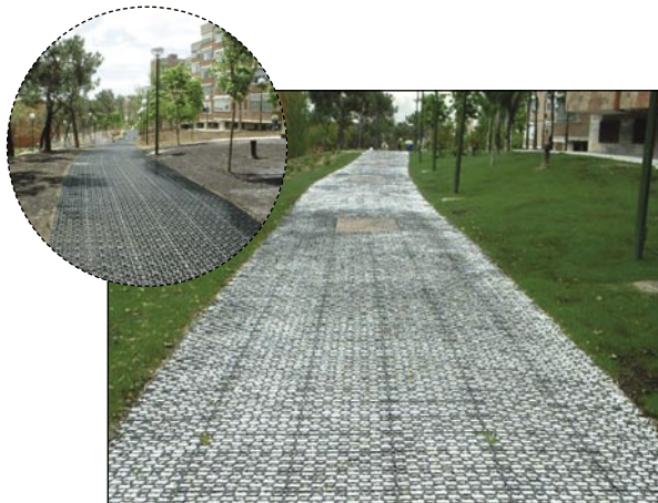
Gravel Cell ® installed for an internal road of a housing development .
