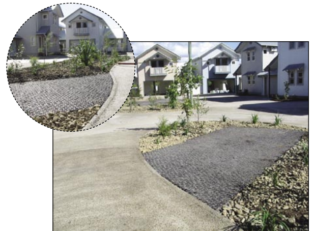
Gravel Cell ® installed for individual car parking lots.
