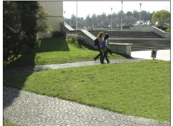
Gravel Cell ® installed for pathways on a university campus.
